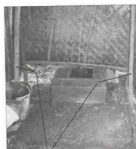
Figure 7.11. Two vertical bamboo support poles one on each side of latrine.
