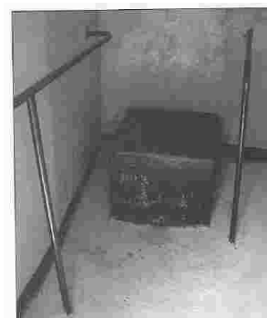
Figure 7.7. Painted rail fixed to floor and walls.
